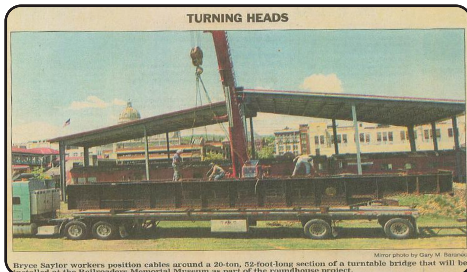
Crane unloading the main frame of the turntable
